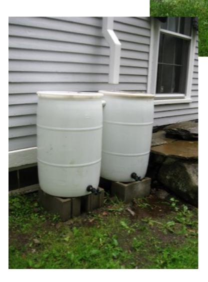
These tanks were elevated off the ground and fitted with garden hose bibs for easy garden irrigation. Rainwater tanks can even be used to charge a drip irrigation system with the right ratio of volume and elevation off the ground.
