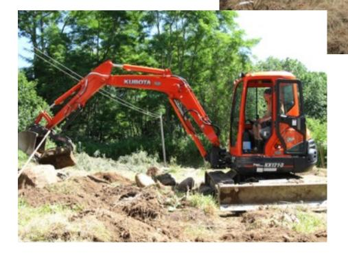
Part of the trick when digging swales is knowing when to stop. It's nice to have someone with an eye that knows when it's deep and wide enough. And that can vary based on steepness of slope.
