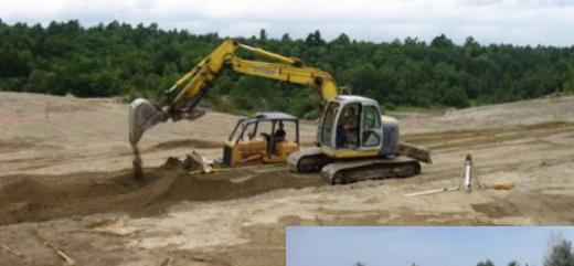
The excavator dug ditches on the inside of each of these terraces which were then filled with wood chips. The soils for this site were very sandy and low in organic matter, and the wood chips acted like a giant carbon-based sponge.
