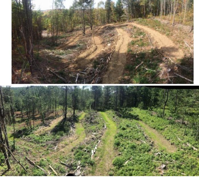
These are the preliminary earthworks for a future chestnut orchard. We were hired to design and manage the construction of these terraces in an existing forest. It was a bit challenging working around stumps and big rocks, but now these earthen shapes will catch and store water in the soil for generations to come.
